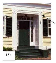
Recessed doorway with thick border molding and columns with corner blocks
